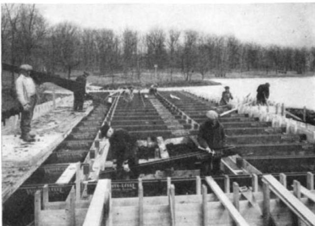
Placing hollow steel sections and (right) light-weight concrete floor, in a new building system
