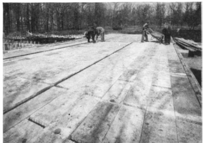
Placing hollow steel sections and (right) light-weight concrete floor, in a new building system
