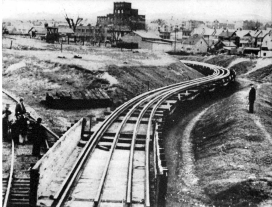
7 Welded rails in transit. When the required number of rails of a given length have been loaded on flat cars, they are dispatched to the point where they will be laid. Long lengths of rails give no difficulty when rounding curves; they bend and straighten as necessary without even being fastened to the bottoms of the cars
