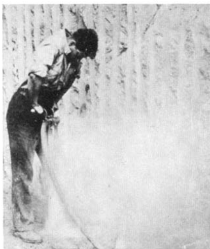
A dangerous concentration of silica dust at left, thrown off in a cloud by a pneumatic drill. On the right a new suction collector carries away all dust
