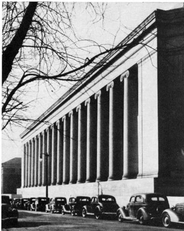
East colonnade of the magnificent new building of the Mellon Institute of Industrial Research at Pittsburgh
