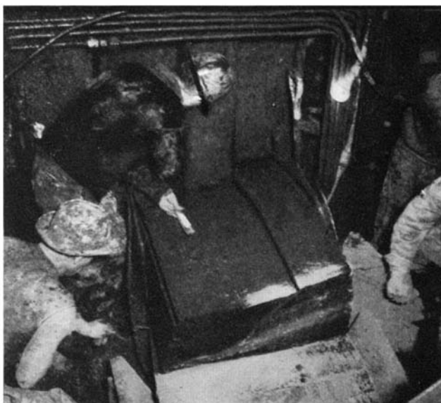
A tough, doughy slab of muck squeezing through an opening in a shield, like tooth-paste from a tube
