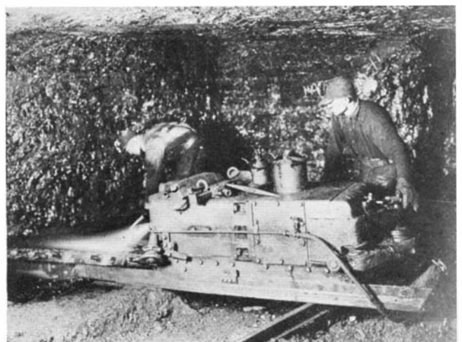
Coal mines constitute another dust hazard and especially at points where machines undercut the coal seam by means of powerful cutting teeth on a flat arm. At the right, this operation is rendered dustless by a spray of water on the cutting arm
