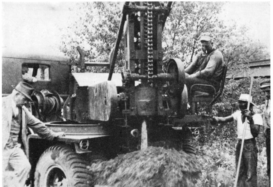
Sinking pole holes with the new motorized augur
