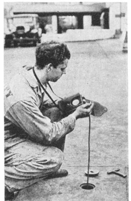
Detecting combustible gas
