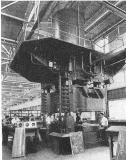
Aluminum alloy parts for airplanes are formed in this hydraulic press
