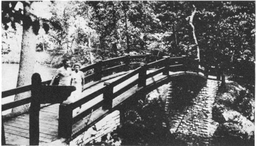
One of the hinged arch bridges discussed below
