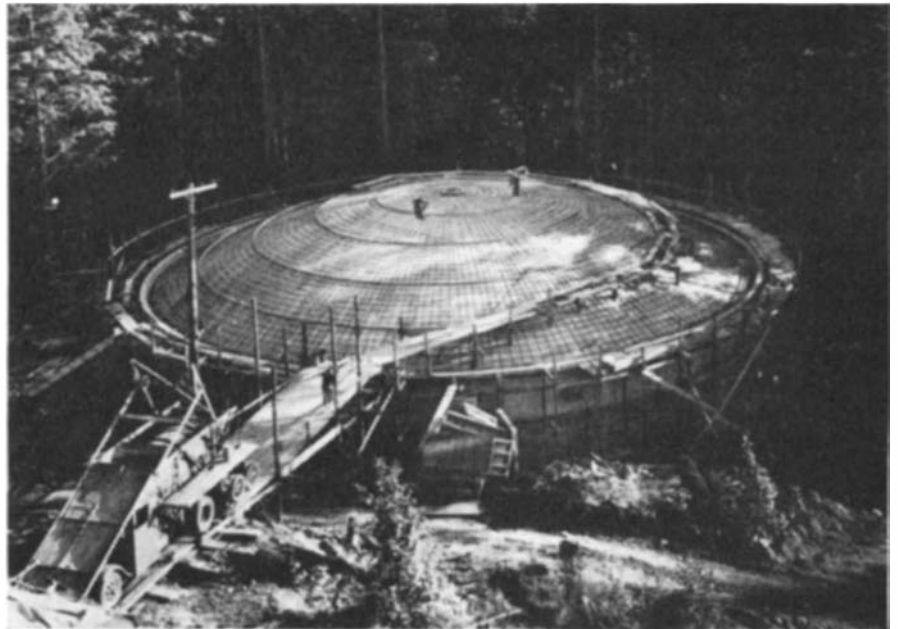
Paper mill requirements necessitated the construction of this huge tank
