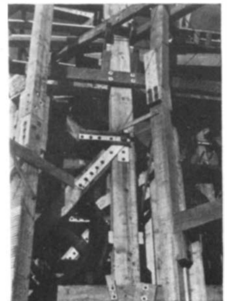
Interconnected steel straps and channels hold timbers together
