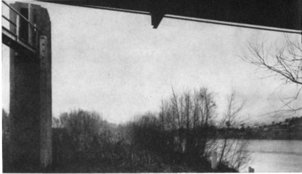
Above is shown one of the stream gaging stations on the French Broad River. At the left: This special radio device announces automatically every two hours whether the river is rising or falling. A similar one broadcasts a record of rainfall
