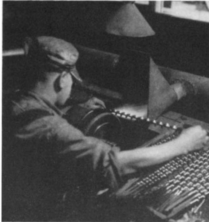
A skilled workman polishes an augur on a grinding wheel
