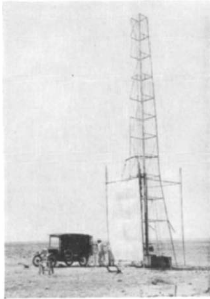
Erection of the 60-foot launching tower formerly employed in the east
