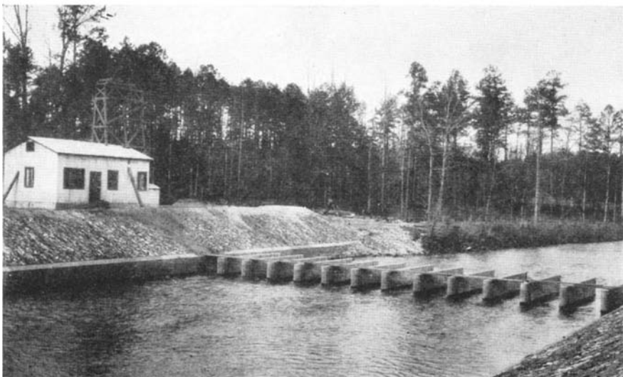
Full-size set-up for studying stream sedimentation
