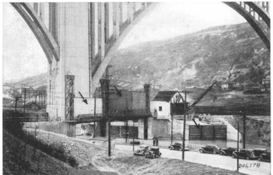
From left to right, the arrows point to the gate in the roadway, the gate over Turtle Creek, and the outlet on the down-stream side of the dam. See the text
