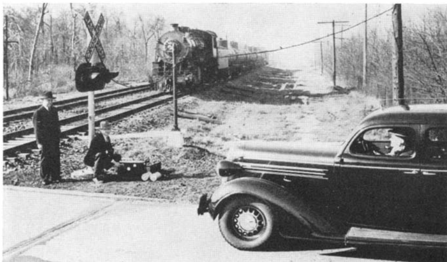
An experimental set-up of the radio railroad crossing warning
