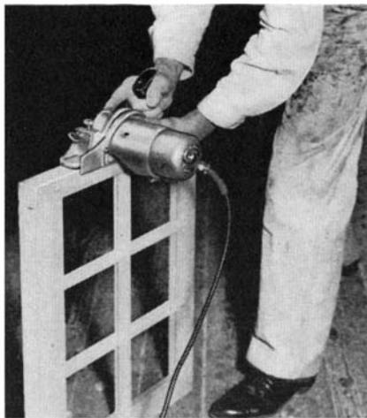
An electrically driven plane speeds up many wood-working operations
