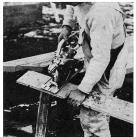
Ripping or cross-cutting may be done with this portable power saw
