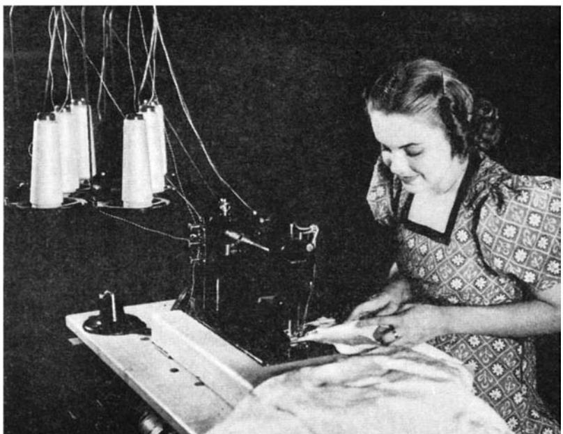
11 Below: Sewing glass cloth with glass thread, making, for the first time in history, a completely inorganic fabric. Fiber glass, made by Owens-Illinois Glass Company and licensees, is fire, vermin and moisture proof, is finding wide use in industry for electrical and thermal insulation, in textile and unspun fibrous forms. Its light weight is an added advantage
