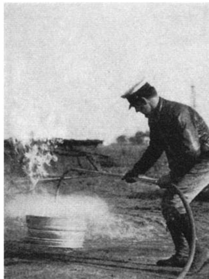
When a stream of water, above, is directed on a gasoline fire, it has little or no effect. When a fog of water, however, is forced through a special nozzle (below) burning ceases almost immediately
