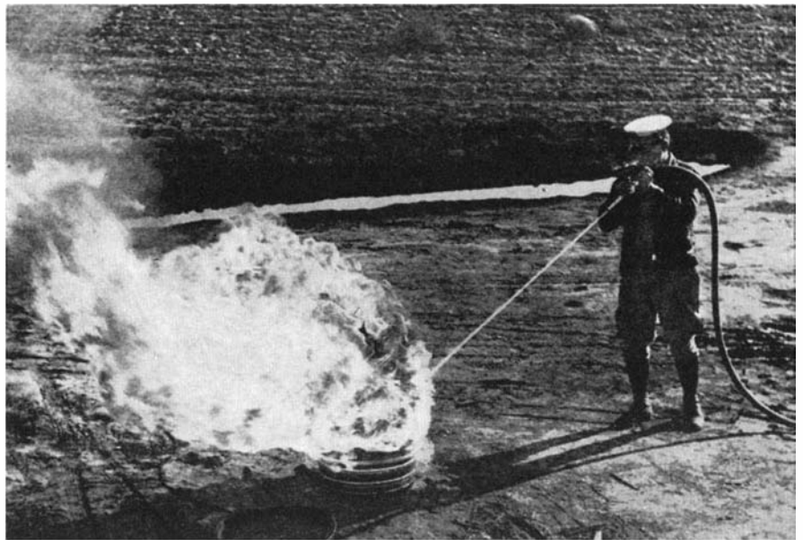
When a stream of water, above, is directed on a gasoline fire, it has little or no effect. When a fog of water, however, is forced through a special nozzle (below) burning ceases almost immediately
