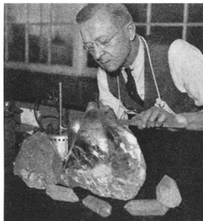
Measuring the quartz crystal prior to cutting it for commercial use
