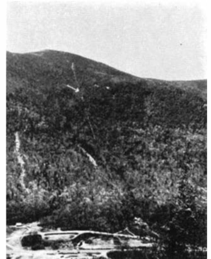
Arrow points to one of tramway supporting towers. Note that scenic beauty of the spot is not marred
