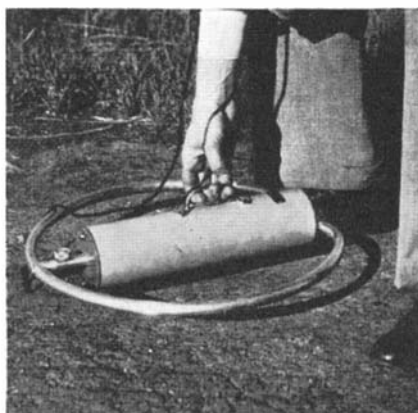
Checking location of a pipe line
