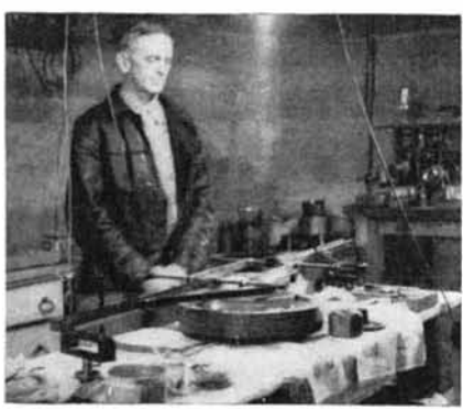
Figure 8: Wells and Hindle rig
