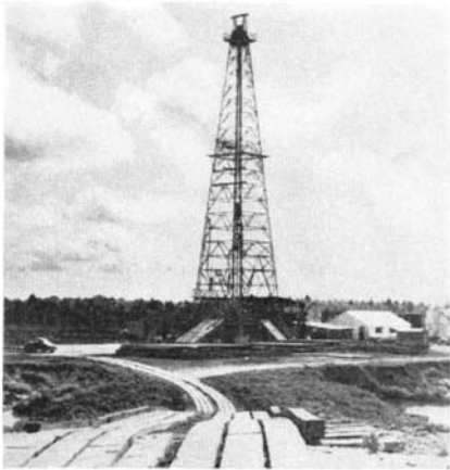
Site of the oil well that has tapped deposits under the Mississippi
