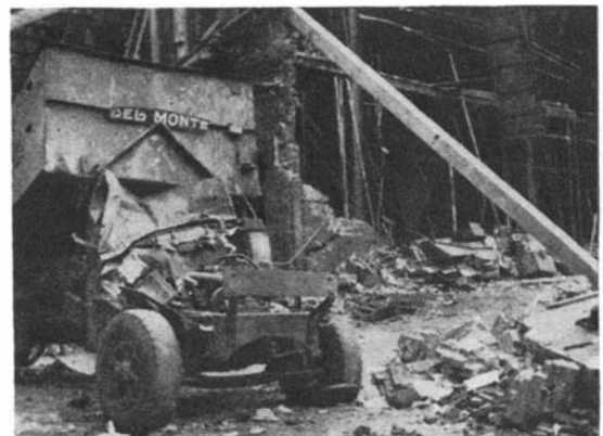
Figure 6: The source of the waves recorded in Figure 7 was a dust explosion in this building
