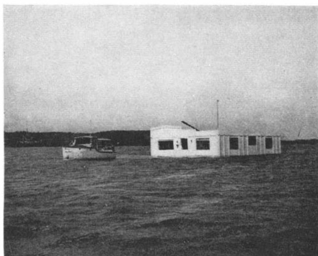
A welded steel house is lowered into the Illinois River and, right, towed to its new home site
