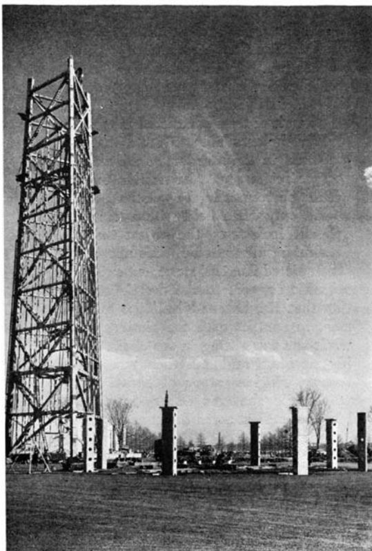
Factory test-assembly to assure fit of lower part of the Perisphere. Below: The Trylon starts upward as Perisphere supports are erected
