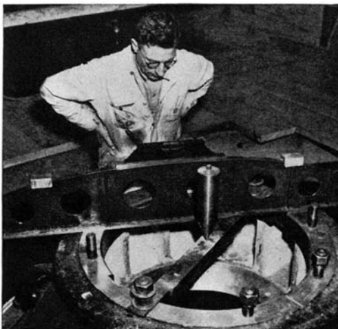
Below: Since the pumps are connected to the motors through long shafts, the scroll cases of the pump units are accurately leveled by a plumb bob and a spirit level on horizontal beam
