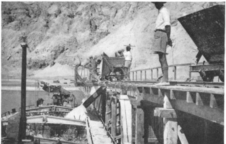
Potash being loaded into a 100-ton barge at the southern pier, immediately below Jebel Usdum, in preparation for towing to the northern end of the lake
