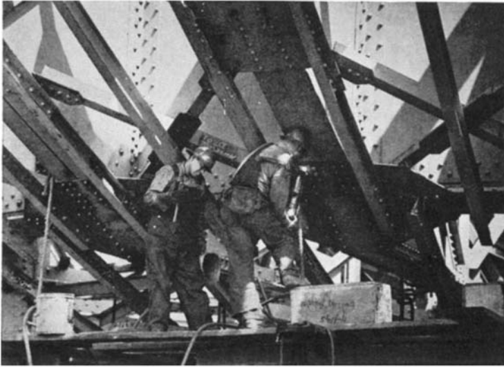
An idea of the size and weight of Perisphere structural steel may be gained from this photograph of rivetting operations under the huge sphere's curve near the base
