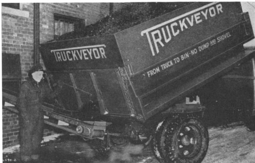
Coal from truck to bin without shoveling or handling
