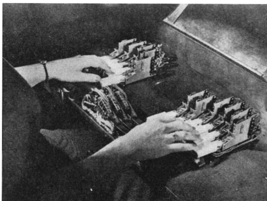
Ten of the white keys each control a speech sound; the eleventh is for volume. The three black keys make the "stop" consonants. The wrist switch changes from consonants to vowels
