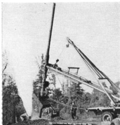
Mushroom-like flames, bursting from a split casing of a gas well, above, were snuffed out, below, after casing was cut with wire rope
