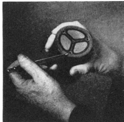
Gas channels in a new cable
