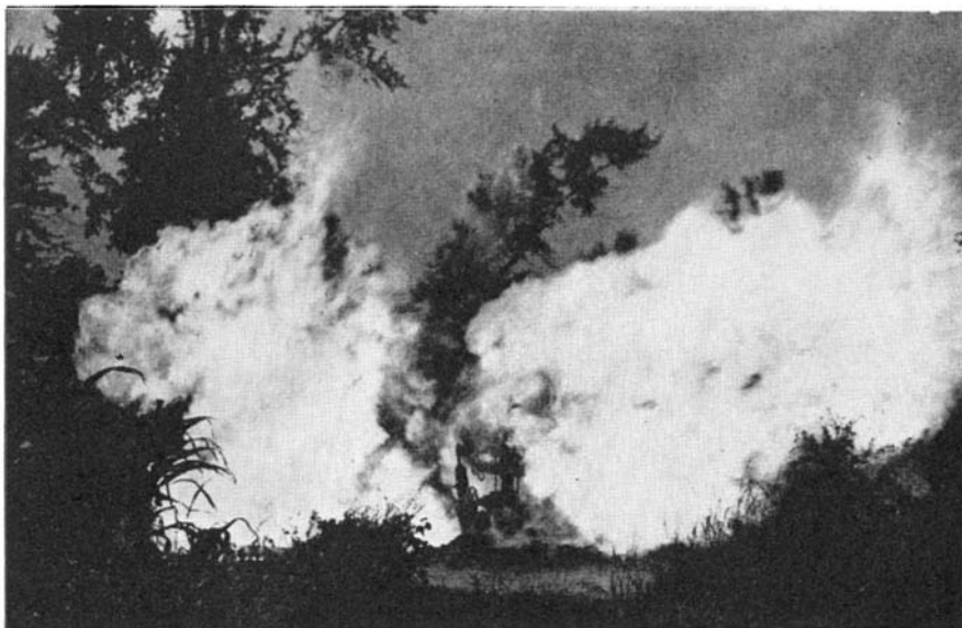
Mushroom-like flames, bursting from a split casing of a gas well, above, were snuffed out, below, after casing was cut with wire rope
