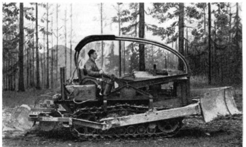
Among new machines in the forests is this combination bulldozer and fire-fighting pump. Two overhead steel tubes protect the driver against branches
