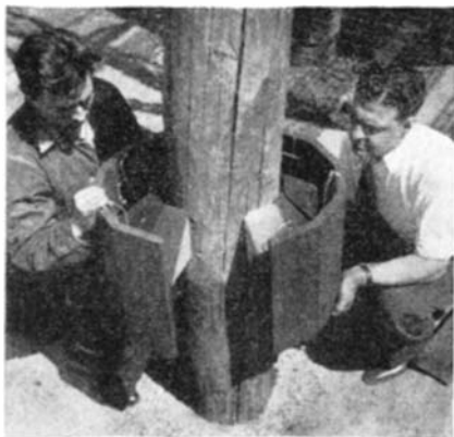
Applying a small section of wooden shield to stop marine borers
