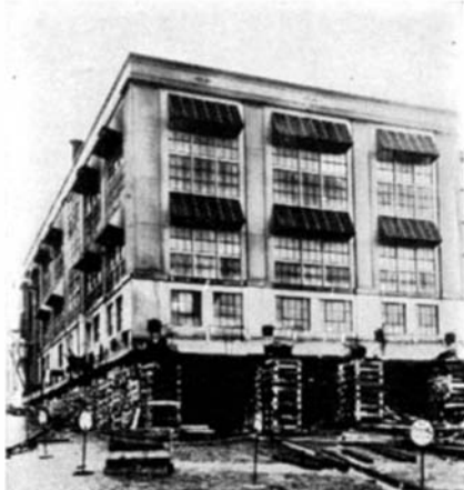
Left: The all-metal office-building ready to be moved. Above: An air view taken during the moving process, showing the difficulties that were encountered
