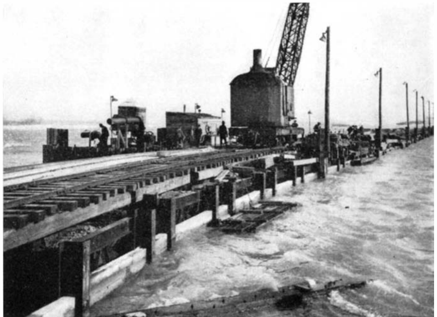
Above: Temporary construction pier that was the base of operations. Below: One of the cells being made ready to be swung outboard and lowered into position
