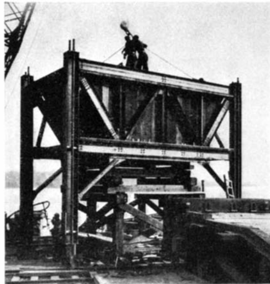
Above: Temporary construction pier that was the base of operations. Below: One of the cells being made ready to be swung outboard and lowered into position
