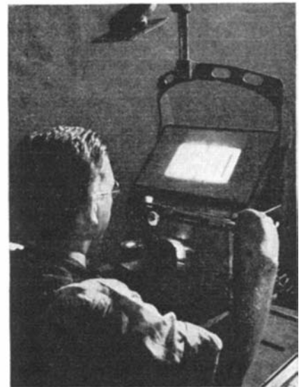
The spectrographic plate is then examined in a microphotometer
