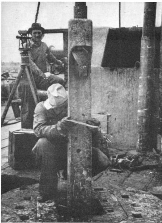
Lining up an Eastman removable whipstock—note slant groove—before lowering into well
