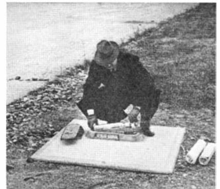
Inserting one of the sodium lighting units used as airport markers
