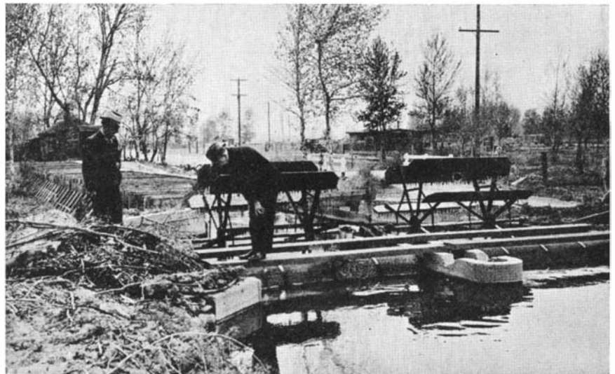
Above and below: Two views of the rotary fish screens in the Yakima River, described below, in which paddle wheels turn the cylindrical barrier screens
