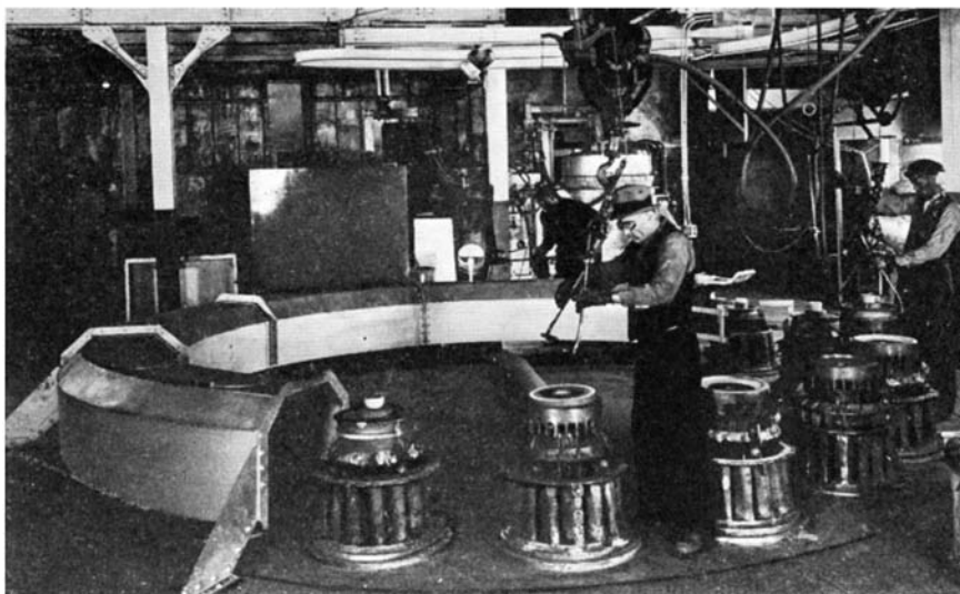
Turntable on which gears are centrifugally cast in 18 dies
