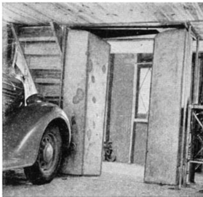
Figure 12: The two massive piers
