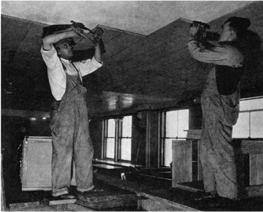
Installation in a school of a Celotex product which effectively absorbs unwanted sounds, prevents reverberations and echos. At right: Johns-Manville sound deadening material being packed into the cushioned floor chairs which are part of a special "floating" construction that efficiently controls all noises
