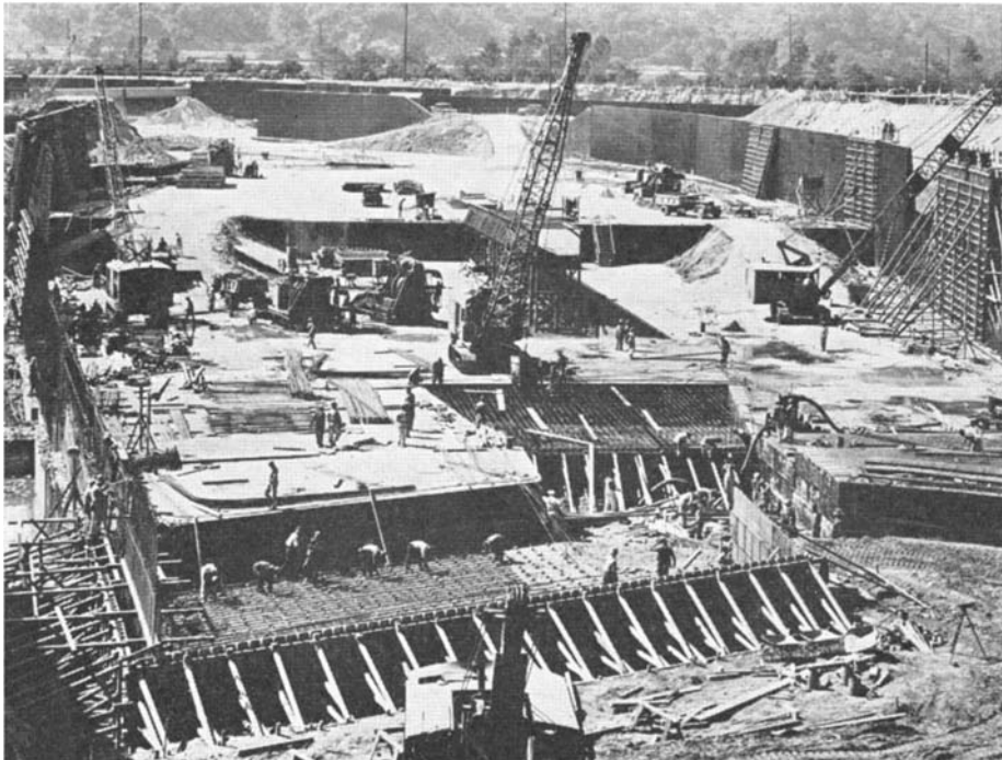
Left: Settling basin at junction of Verdugo Wash and Los Angeles River, showing baffles (foreground)
