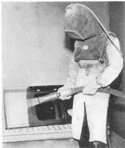
Sand blasting for reclamation
