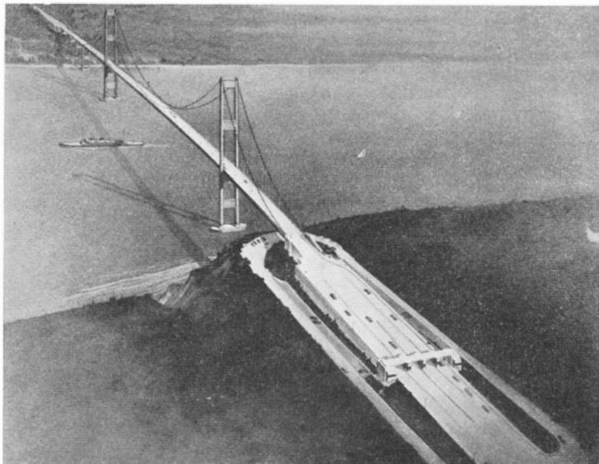
As the new bridge will look when completed. Note "lookout point"
