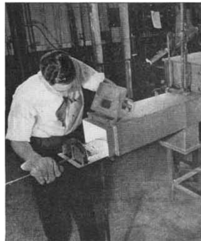
Removing a block of air-hardened steel from heat-treating furnace
