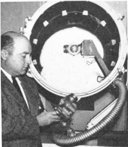
The small object held in the hand is the complete light-source unit of the 25-million-candlepower searchlight shown in the background
