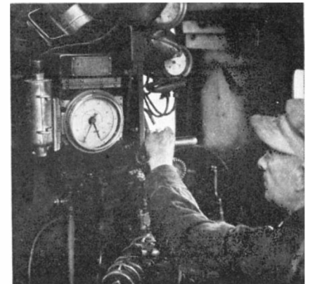
Location of the Loco Valve Pilot in the cab of a steam locomotive
