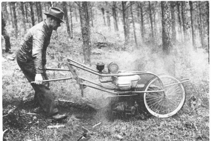
Demonstrating the fire-trench digger described above
