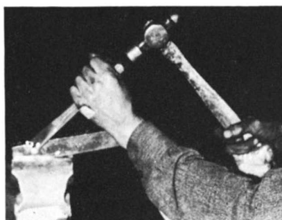
Beryllium-copper tools find use near explosives because they won't spark, will easily cut cold-rolled steel, below
