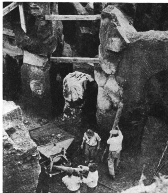
Workmen with dump cars of earth and debris to be removed from beneath the arena
