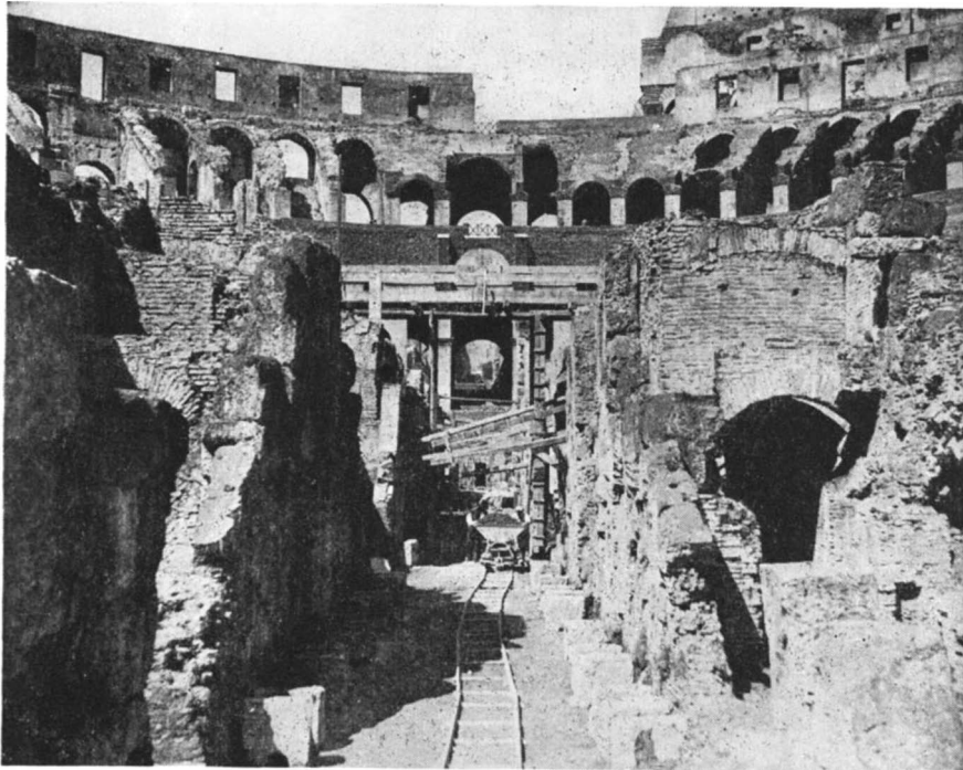
Laborers trundling a dump car along a light track 20-odd feet below the level of the ancient arena. Through these same passageways howled the lions of old Rome
