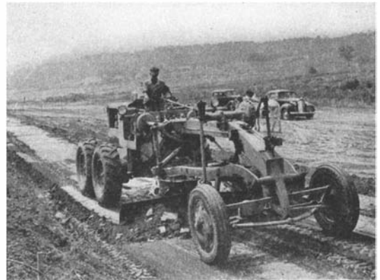
One of the many rubber-shod pieces of construction equipment used
