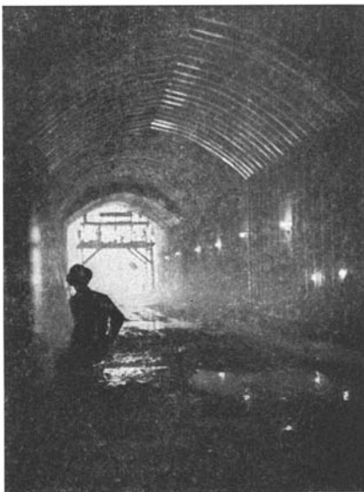
Steel supports inside one of the re-bored and widened old tunnels
