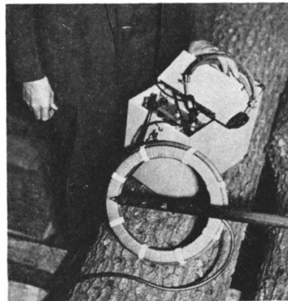
Exploring coil and detector box of device for locating hidden metal
