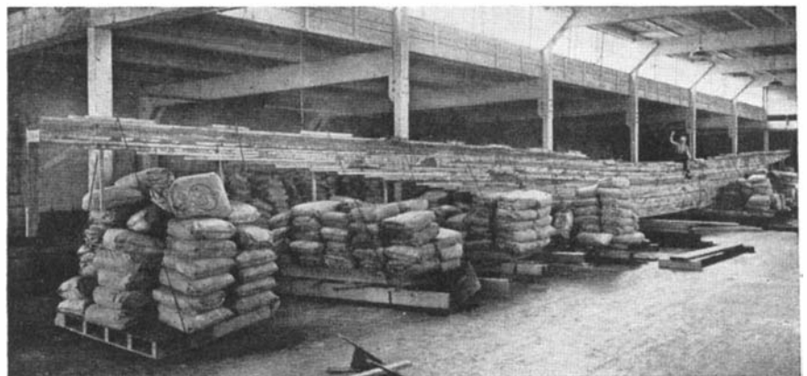
There are 3780 board feet of lumber in this 8791-pound beam
