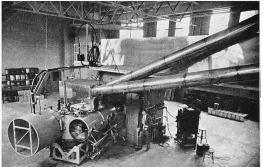
The same cyclotron viewed from the power supply house on the balcony. Nearer cylinder is a vacuum chamber down which particles finally speed
