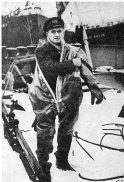
Designed for seamen, this life-saving suit is quickly closed by means of a "zip" fastener
