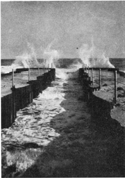
At left: Typical sea water intake which will conduct water to settling basins, the first step in production of magnesium from the sea
