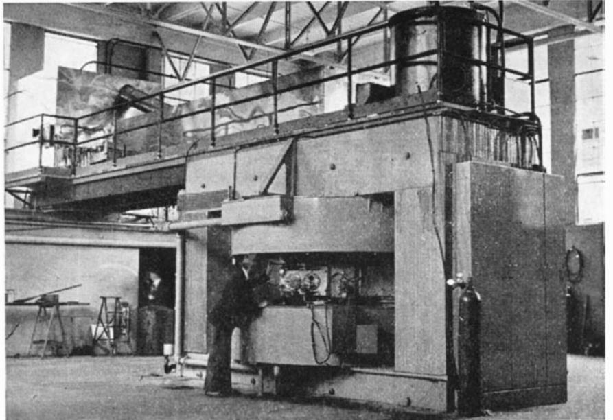
The 220-ton cyclotron at the University of California. The big chunky rectangle, with vertical pole-pieces in its middle, is the huge magnet. Between these pole-pieces is the main, "business" part of the apparatus, the circular vacuum chamber containing two electrodes, also the space where projectile particles are speeded up. Power source is on balcony
