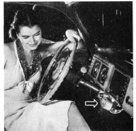
Arrow points to battery condition indicator on motor-car dash
