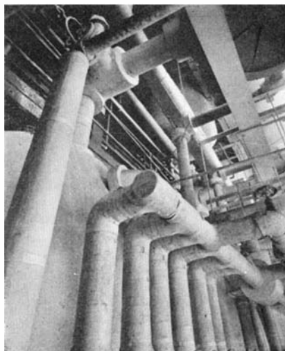
Stills used in making synthetic camphor from CO 2 and ammonia
