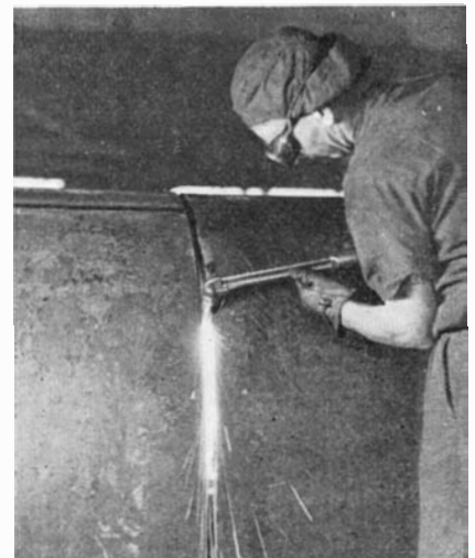
Steel is cut cleanly, rapidly with the oxy-acetylene torch
