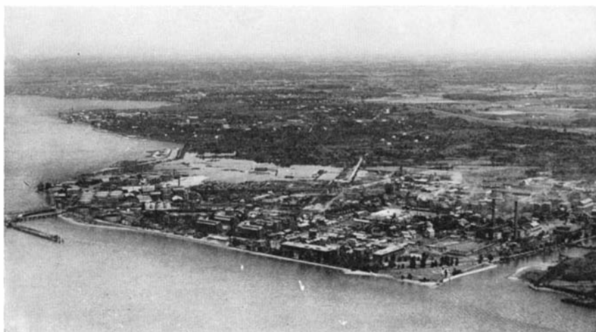
Plant where several well-known organic chemical products are made — du Pont plant at Deepwater, New Jersey. Note many buildings
