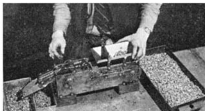
Steps in salvaging rivets. Lower left: Sorting for diameter with sifter. Above: Sorting for length. Below: Separating round-heads from flat-heads
