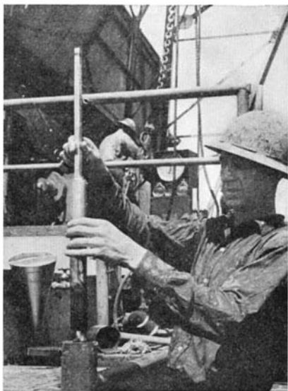
Checking specific gravity of mud returned from circulation
