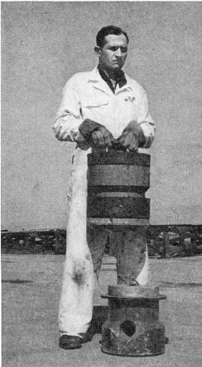
The wooden blocks that are used when concreting a well
