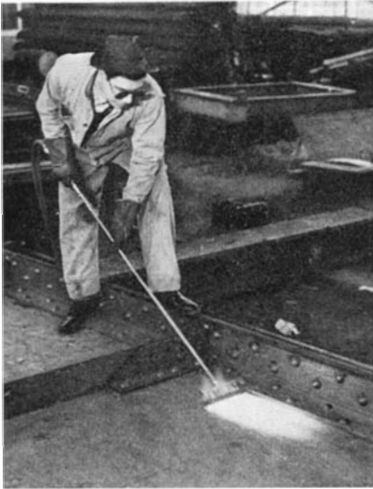
Oxygen flame rapidly cleans steel surfaces for painting
