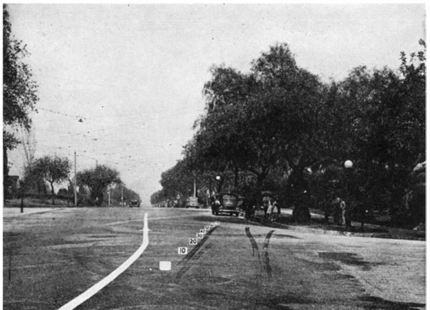
Skid marks 60 feet long, left by a car at the scene of an accident. Marker boards are shown laid on the pavement at ten-foot intervals by the police
