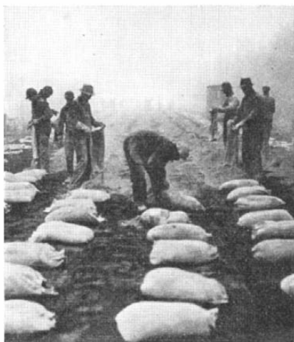
Above: Spreading cement for resurfacing a dirt road. Below: Cutting the cement into the dirt
