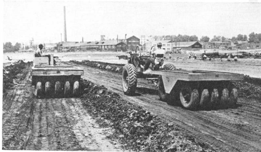
Multiple pneumatic tires replace the iron barrel of the steam roller
