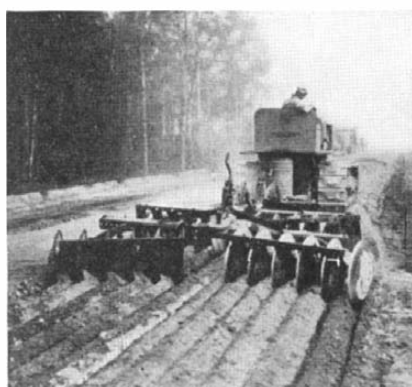
Above: Spreading cement for resurfacing a dirt road. Below: Cutting the cement into the dirt
