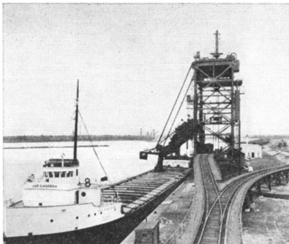
The kick-back trestle of the new dumper, and, beyond, the loaded-car and empty-car yards
