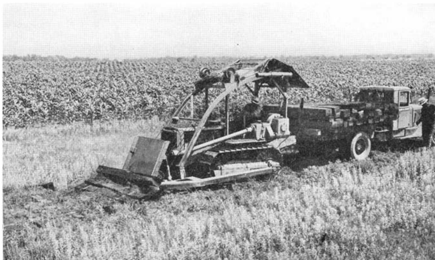
Mobile unit salvages ties from an abandoned railroad
