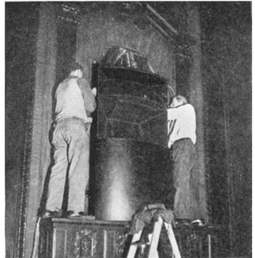
One of the large speaker units located in the theater balcony
