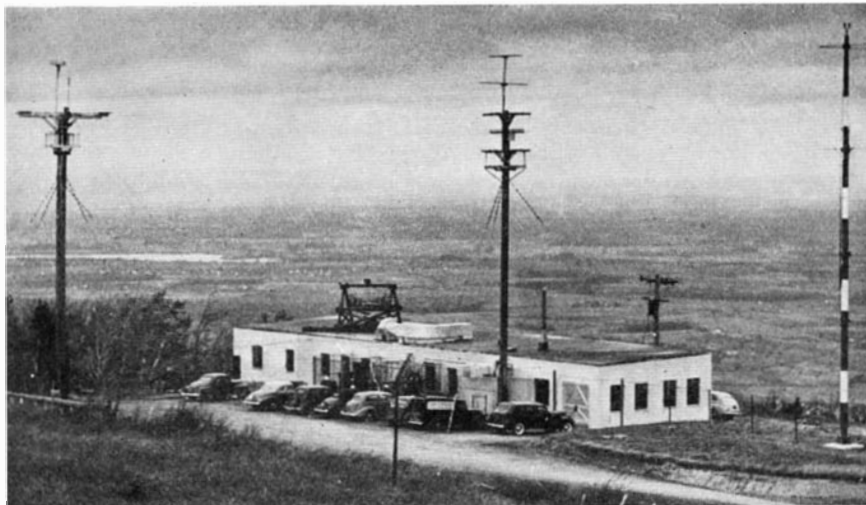
W2XOY, General Electric station near Schenectady, New York, used for both television and FM. At right is frequency-modulation antenna
