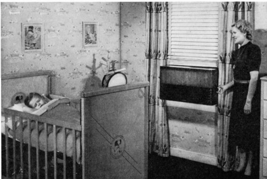
Window unit provides warm or cool conditioned air
