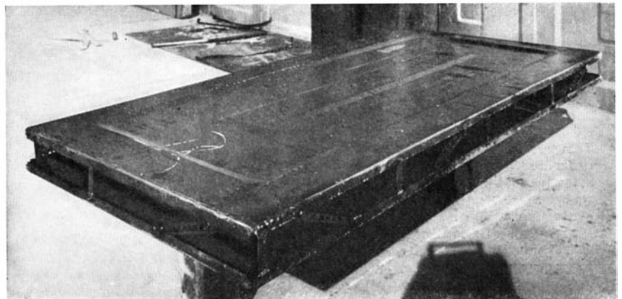
A building block of welded steel
