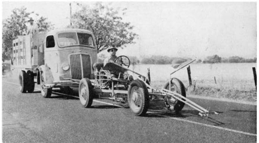
Applying white lacquer and glass beads to a traffic stripe
