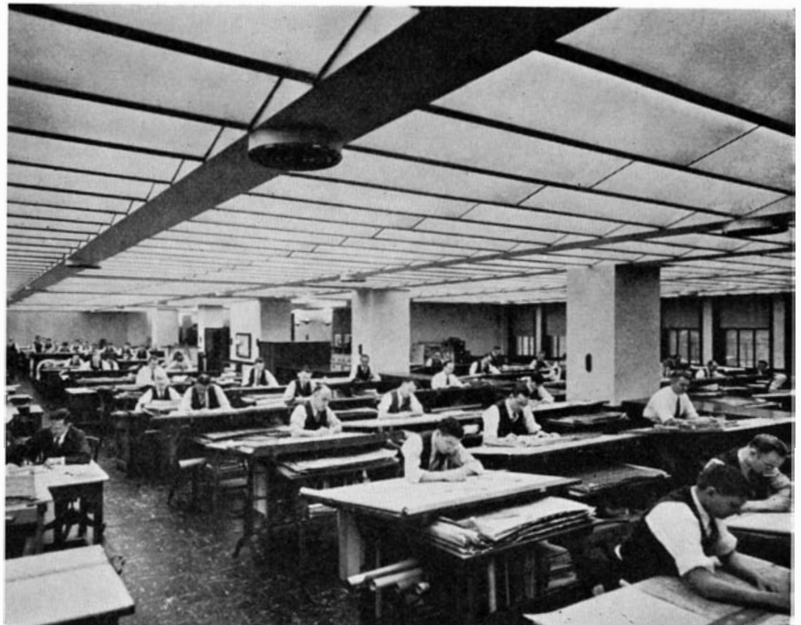
Fluorescent tubes in angular reflectors illuminate a drafting room
