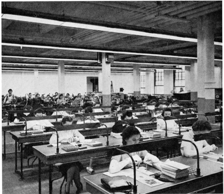
Overhead fluorescent lighting, plus individual units on assembly benches
