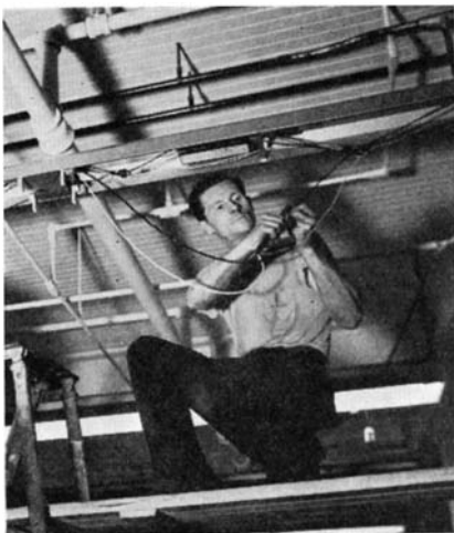
Installing industrial lighting fixtures for fluorescent tubes
