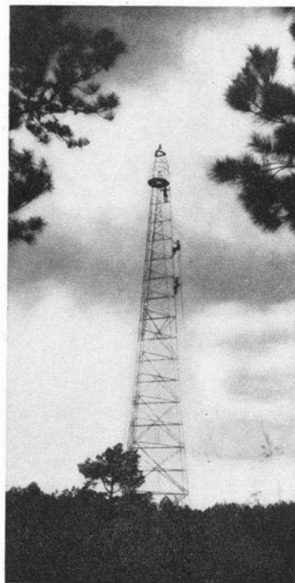
Figure 4: Steel towers like this can be used for triangulation on land, but cannot be set at sea, hence, less direct means are used
