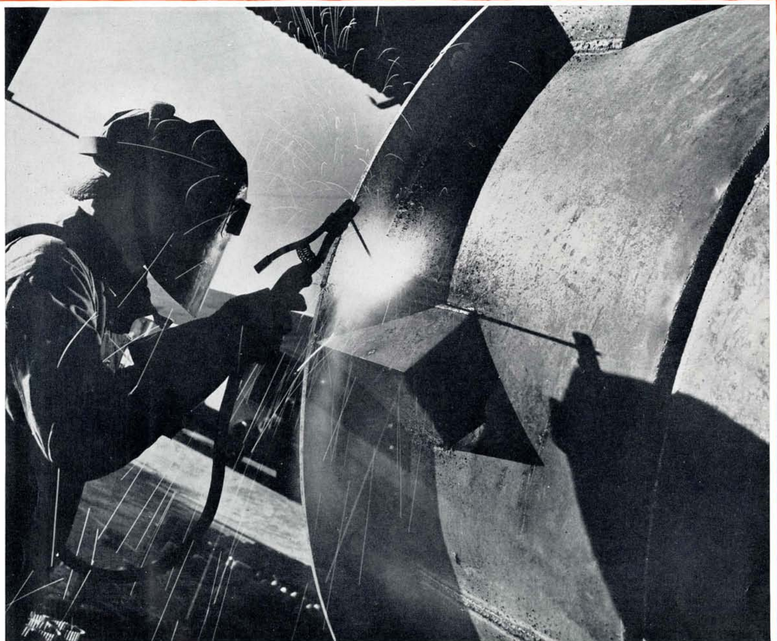
Welding Breaks Bottlenecks
