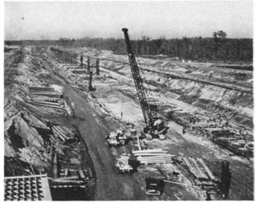
Construction view of longest earthen dam—the Santee—in the United States
