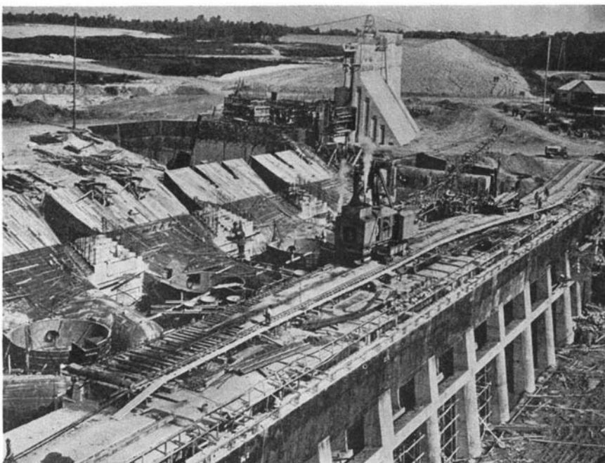
Retaining wall, turbine construction, discharge end of draft tubes
