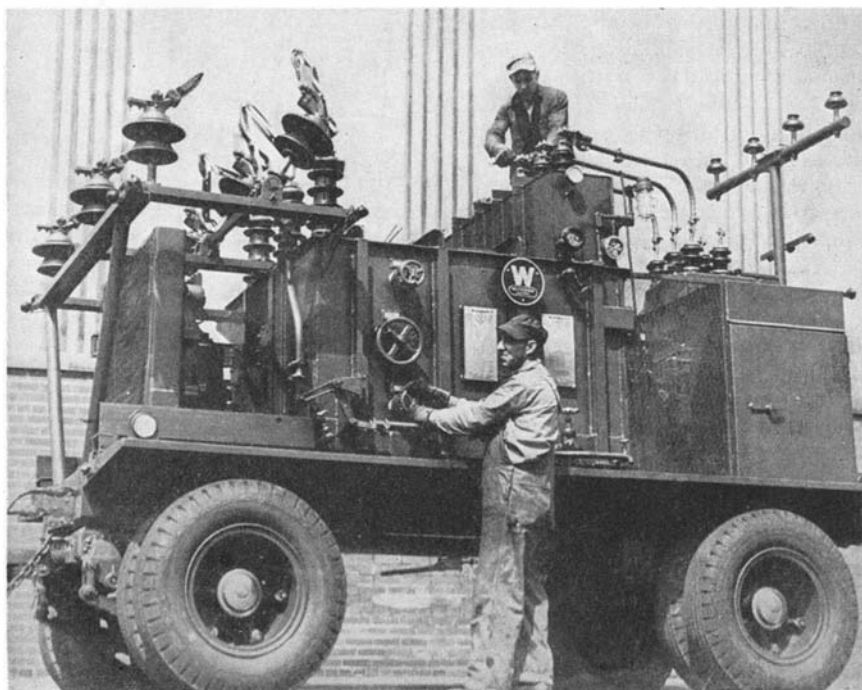
A complete transformer substation on wheels
