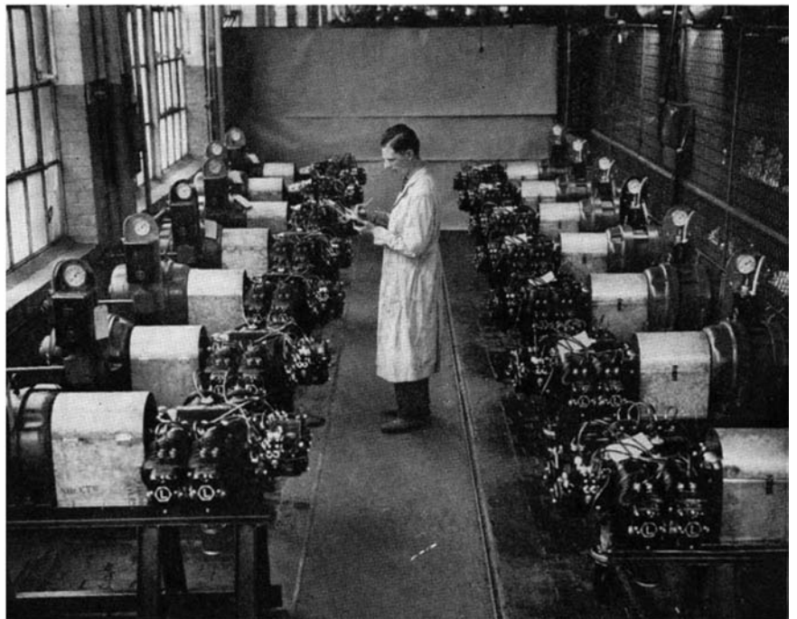
Electrical run-in stands test 50 airplane engines daily
