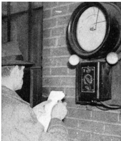
Typical installation in a boiler room of solu-bridge control unit
