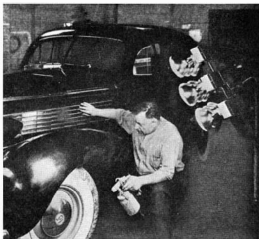
Even small shops that do automobile body repair jobs find profit in portable radiant heat units for drying paint patches
