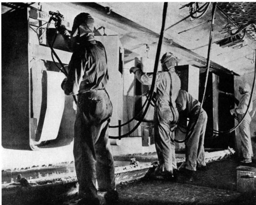
Unused paint falls into vats, is salvaged for further use
