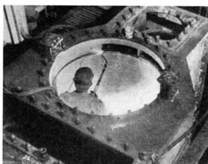
How welding was used to repair cylinder walls in ship power plants without removing engines. Below: General view of a welder at work. Above: Welding into place a cast section shaped to fit the break. Above, left: A completed weld after boring
