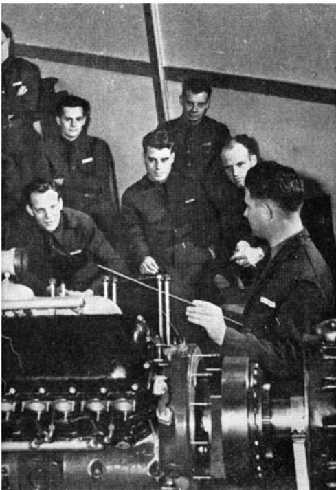
a partially dismantled Allison engine
