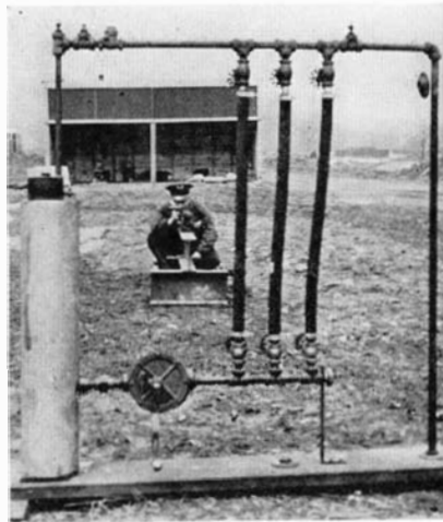
Above: Testing bullet-sealing hose with .50-caliber machine gun. Left: Despite holes, hose held fuel at 10-15 pounds pressure
