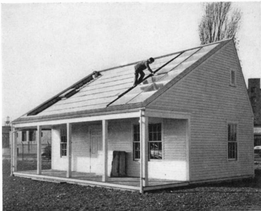
Sun laboratory where the plan to heat a building by solar energy is tested
