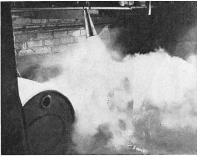
A storage room packed with inflammable materials is protected against fire by a carbon dioxide system. At left,
