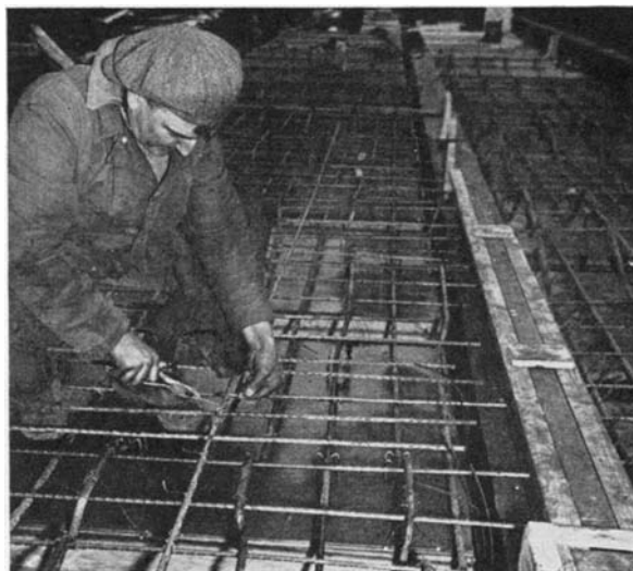
More than a million wired joints, each twisted with special anti-Axis gusto, went into preparation of framework
