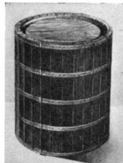
Right: One of the new barrels made with plywood staves locked in place with steel straps. Above: One of the containers in collapsed form for re-shipment
