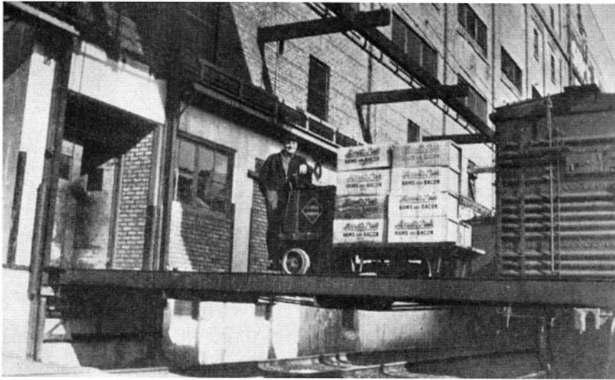
Bridge in lowered position for crossing railroad tracks
