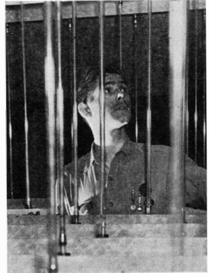
These ultraviolet ray lamps will help to purify the incoming air in ducts
