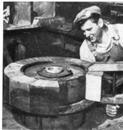
Two views of the method of applying a new wooden tire for trailer use
