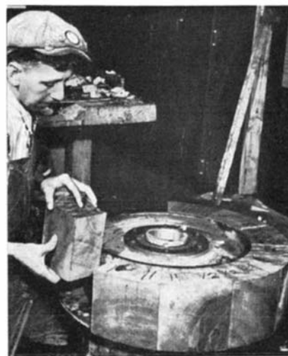
Two views of the method of applying a new wooden tire for trailer use
