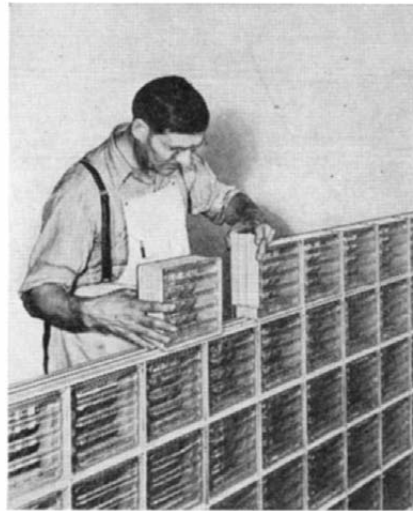
Setting up a portable glass wall
