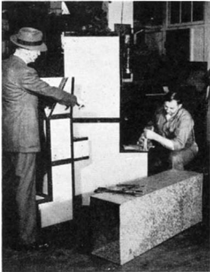
Air ducts of composition board, with replaced metal duct in the foreground
