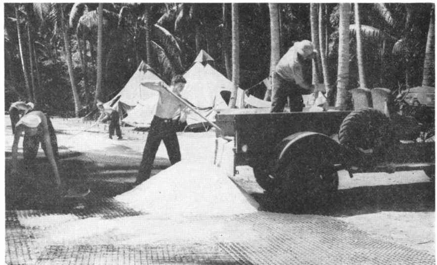
On "Island X" Seabees lay steel mesh on sand for road foundations, then camouflage mesh with finely ground coral, which eventually cakes into hard surface
