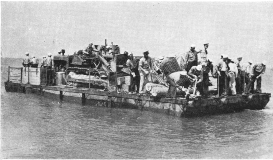
A powered pontoon landing barge, loaded to capacity with men, machinery, and tons of many kinds of materials, chugs its way toward shore in practice maneuvers
