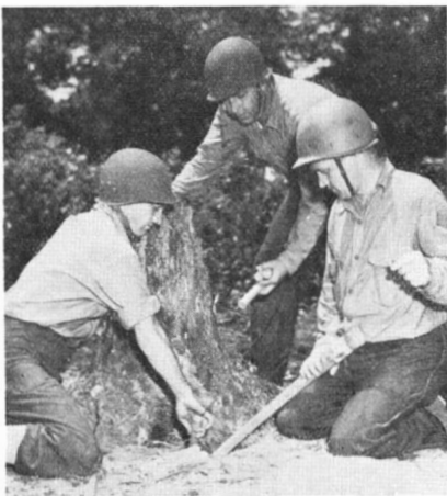
The dynamite crew sets a charge
