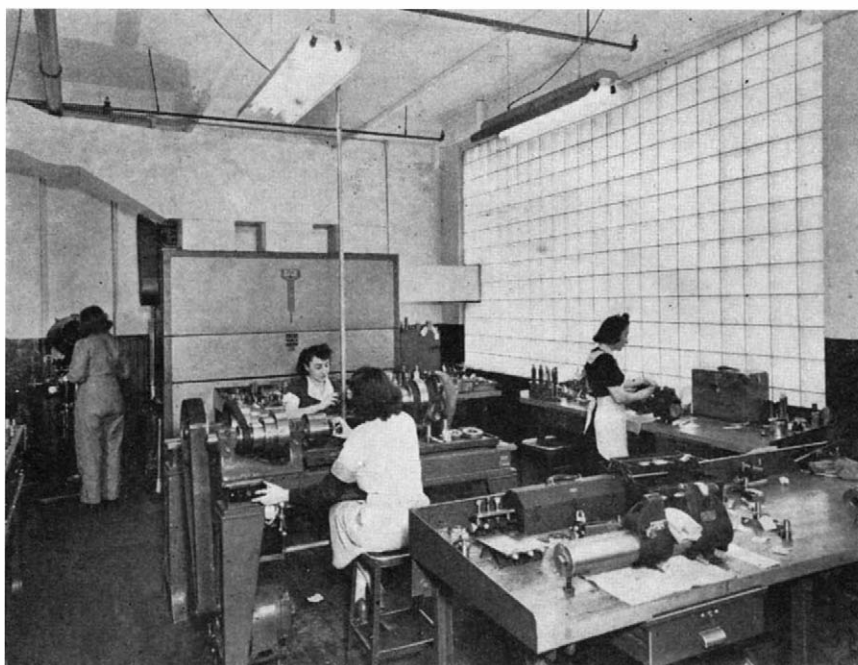
Wall and floor duct installation in a precision tool plant
