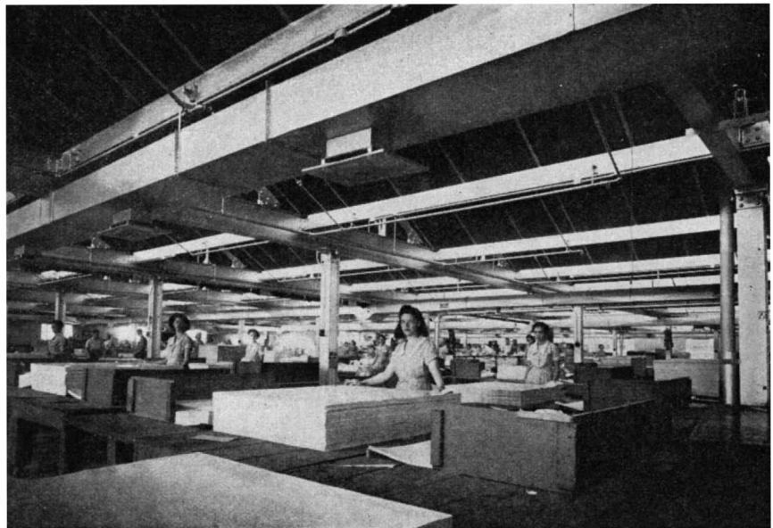
Overhead ductwork in a paper sorting and cutting department
