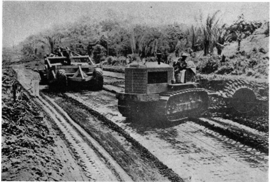
Progress on a road construction project in Costa Rica
