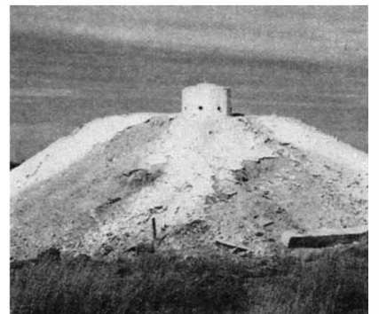
Concrete housing for bomb microphone
