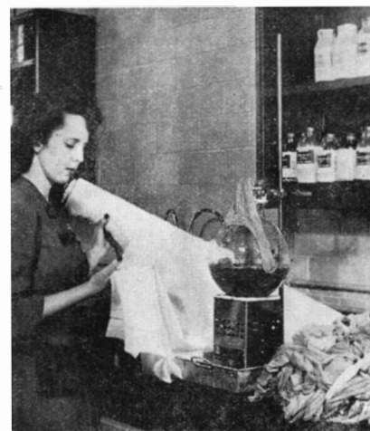
Nylon reversion on a laboratory scale
